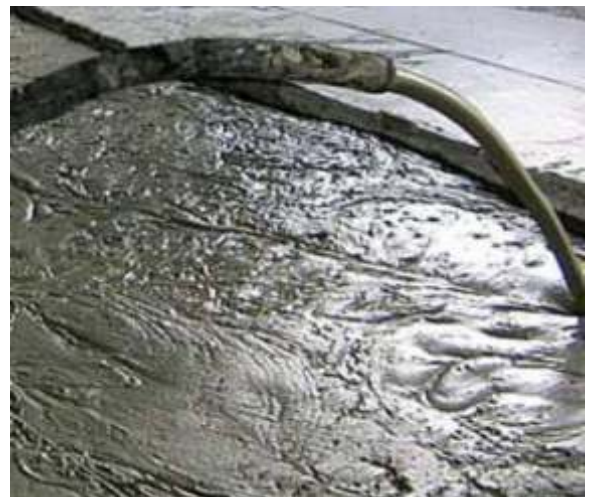
Pos. 10 Filling of ECOLIT lightweight screed
